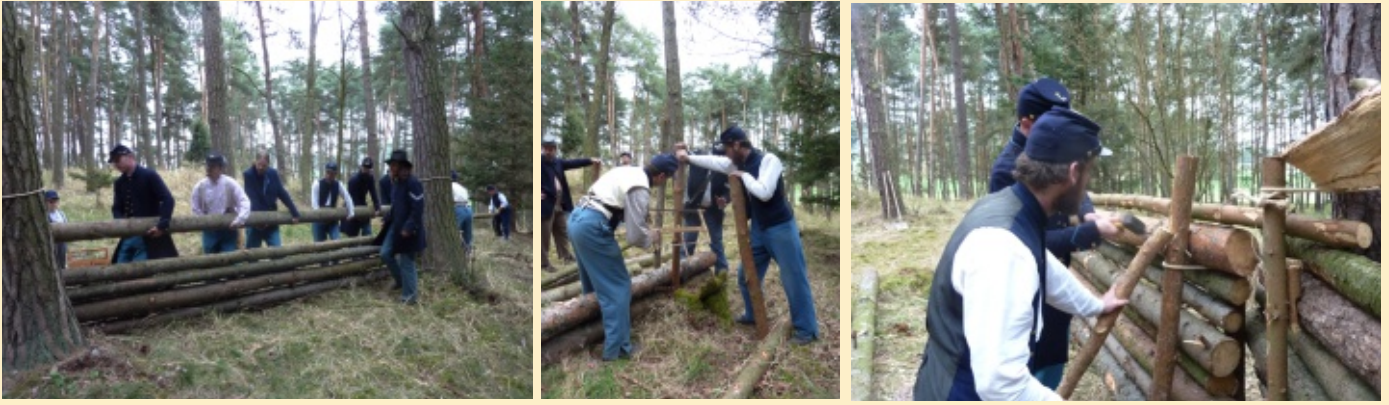
Building of trial breastwork in spring 2014
